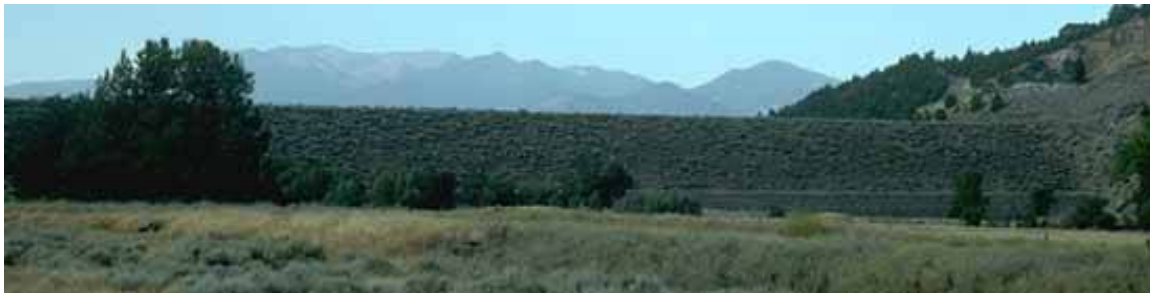
Figure 4. Dwinnell Dam has blocked upper Shasta River spawning areas since 1928, loses 50% of the water it holds to evaporation and leakage (NAS, 2003) and contributes to water quality problems in the Shasta River.
