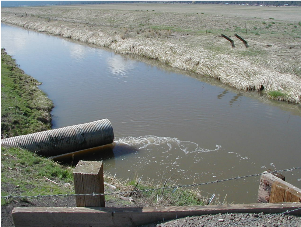
Figure 6. Lost River at Johnson Road with agricultural tailwater pouring in from the culvert at left. Photo by Bill Hobson of the NCRWQCB.
