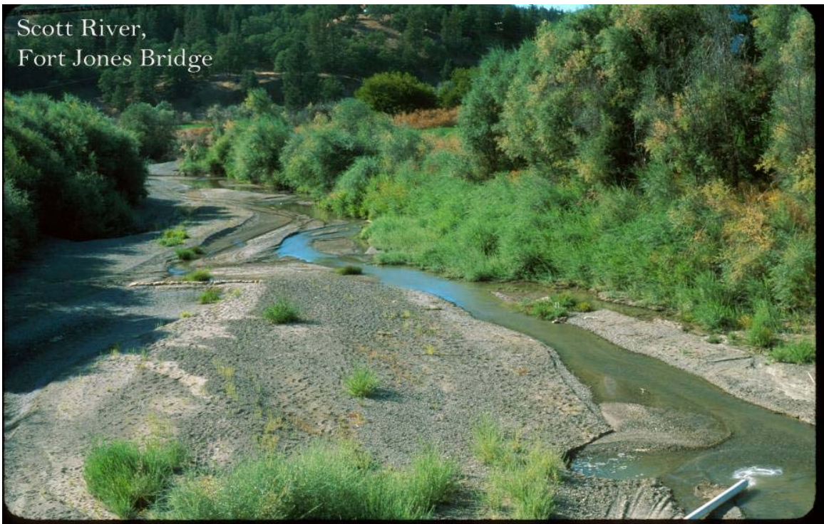
Figure 8. Scott River at Fort Jones Bridge looking downstream. Note streambed is comprised of mostly sand. Photo from KRIS taken by Michael Hentz. 2002.
